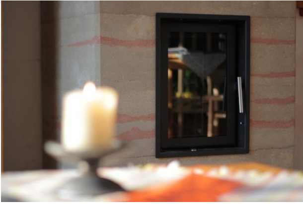
Fig. 1. Luxury rammed earth fireplace prepared by the authors.
